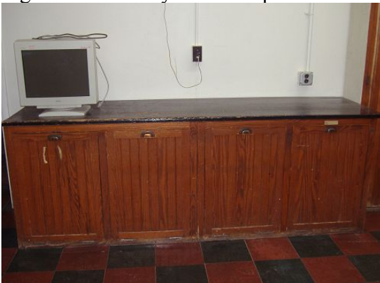
Figure 3: Remaining cabinets, on second floor.
