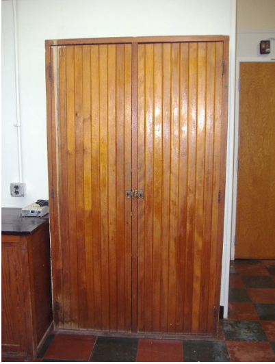
Figure 4: Remaining Cabinet, on second floor.
